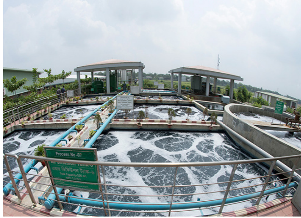
Figure 3: Effluent Treatment Plant
