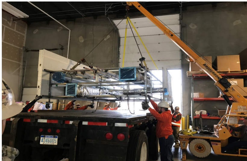
Figure 5: MEP Rack Systems Loaded on the Semi-Truck at the Fabrication Shop
