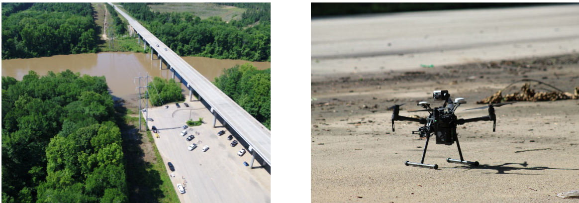
Figure 1: (a) Test bridge and (b) DJI M10 RTK UAS used in the inspection
