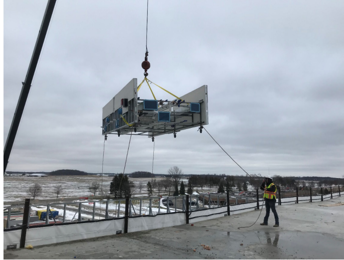
Figure 6: MEP Rack Systems being lifted at Site
